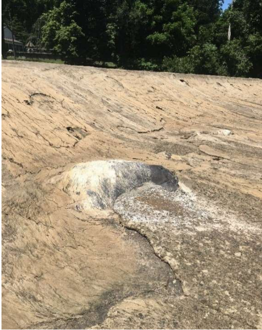
Photograph 5: Boulder embedded in concrete spillway.
