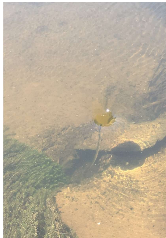
Photograph 8:1 Vortex Forming in Impoundment due to Leakage.
