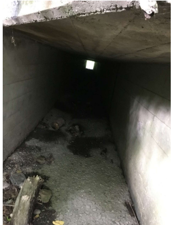
Photograph 12: River Left Sluiceway under Culvert for Abutment (Left) and Road (Right).
