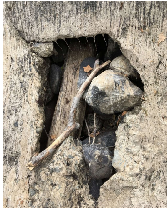
Photograph 6: hole in concrete spillway revealing timber.
