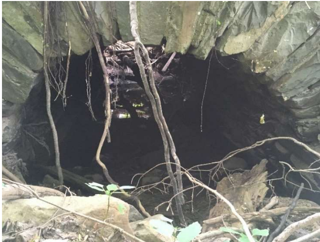
Photograph 12: River Left Sluiceway under Culvert for Abutment (Left) and Road (Right).
