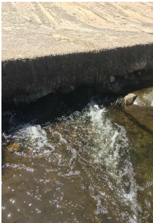
Photograph 7: Leakage under Spillway Downstream of Dam.
